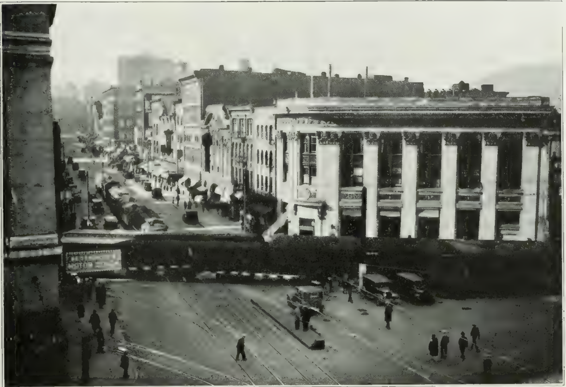
C.P.R. Carrall Street Level Crossing.
